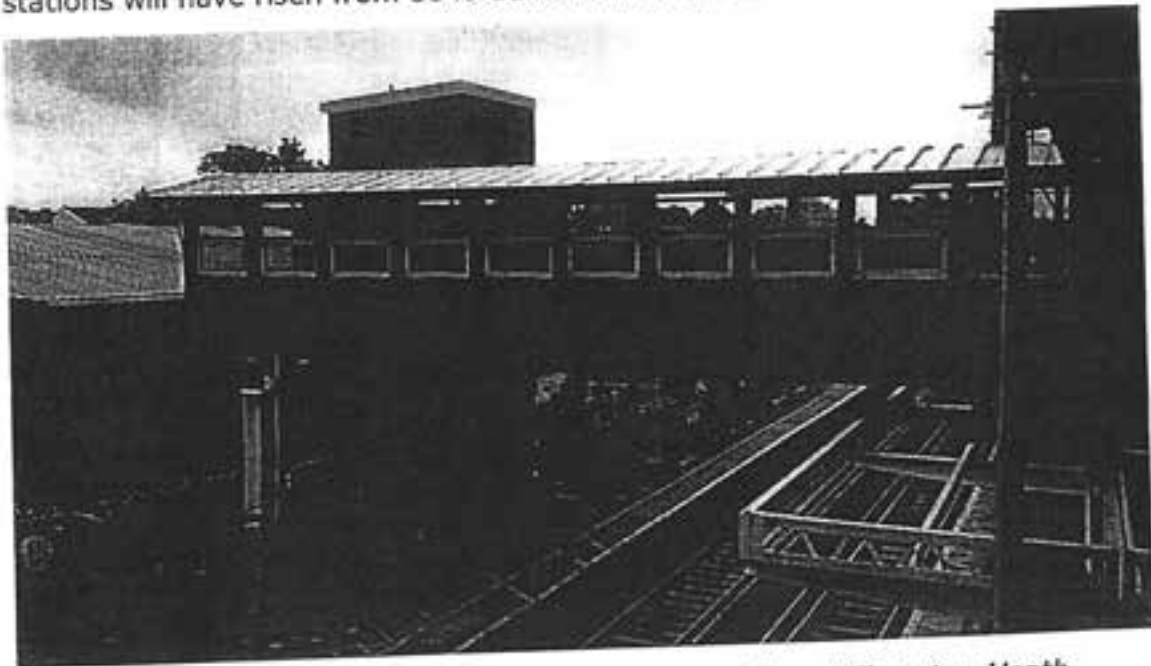
Figure 12: Access for All lift scheme under construction at Thornton Heath
