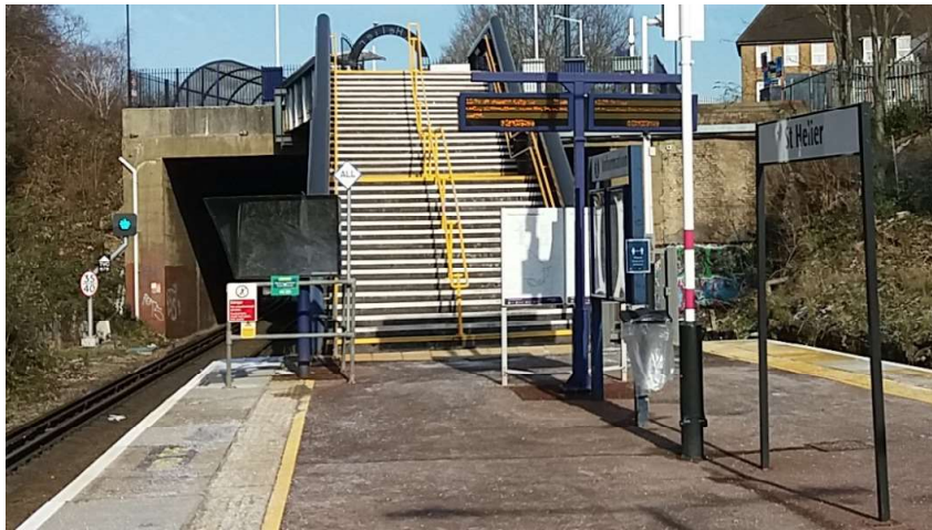
Fig 2: St Helier station, the nearest station to St Helier Hospital – access to platforms via stairs only
