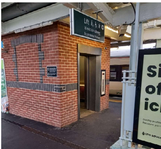
Fig 12: lift at Balham station
